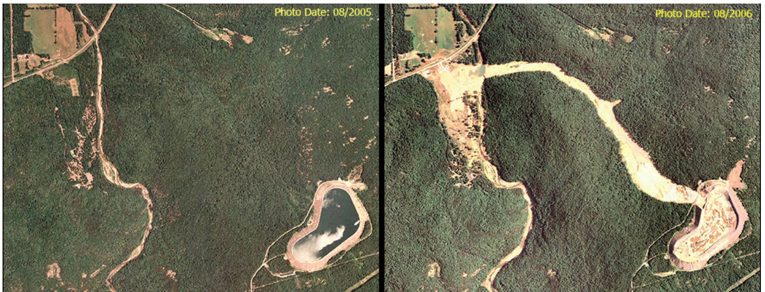
Figure 15 . Taum Sauk Pumped Hydro Catastrophic Drainage (Before and After)
