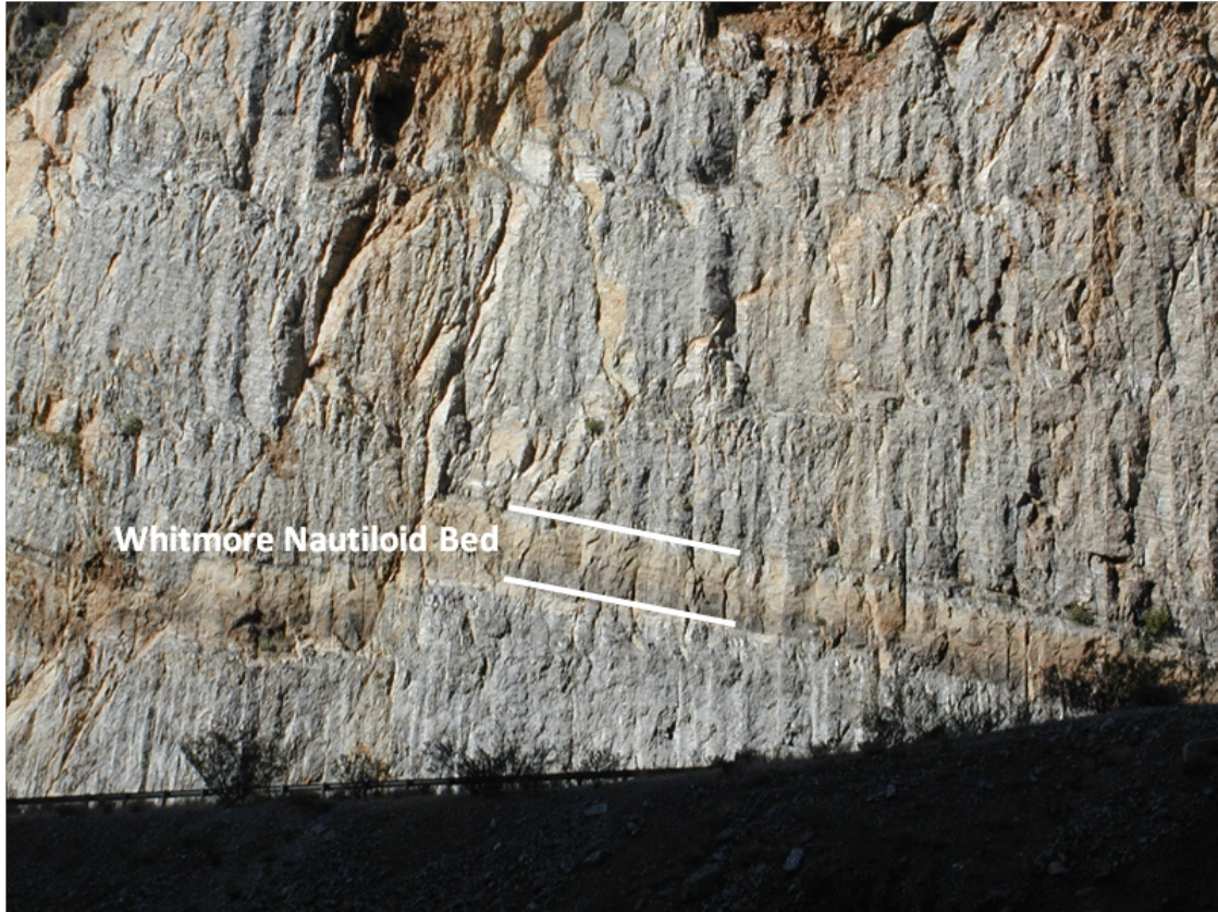
Figure 9. Contacts of WNB at Virgin River Gorge. The roadcut provides a fresh exposure of WNB and the guard rail in the lower portion of the picture provides scale.
